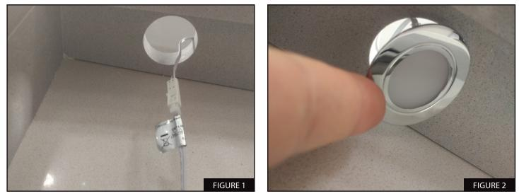
Step 5. Feed the main cable through the LED hole from the top allowing some slack for connecting the other components.
